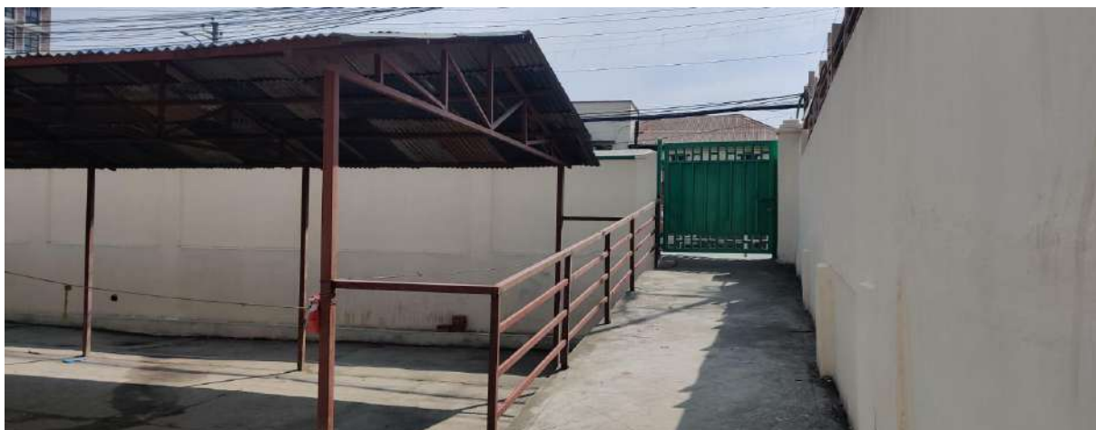
Figure 50: Newly constructed Emergency Exit.
