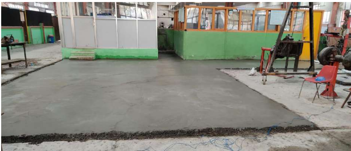
Figure 56: PCC works on progress.
