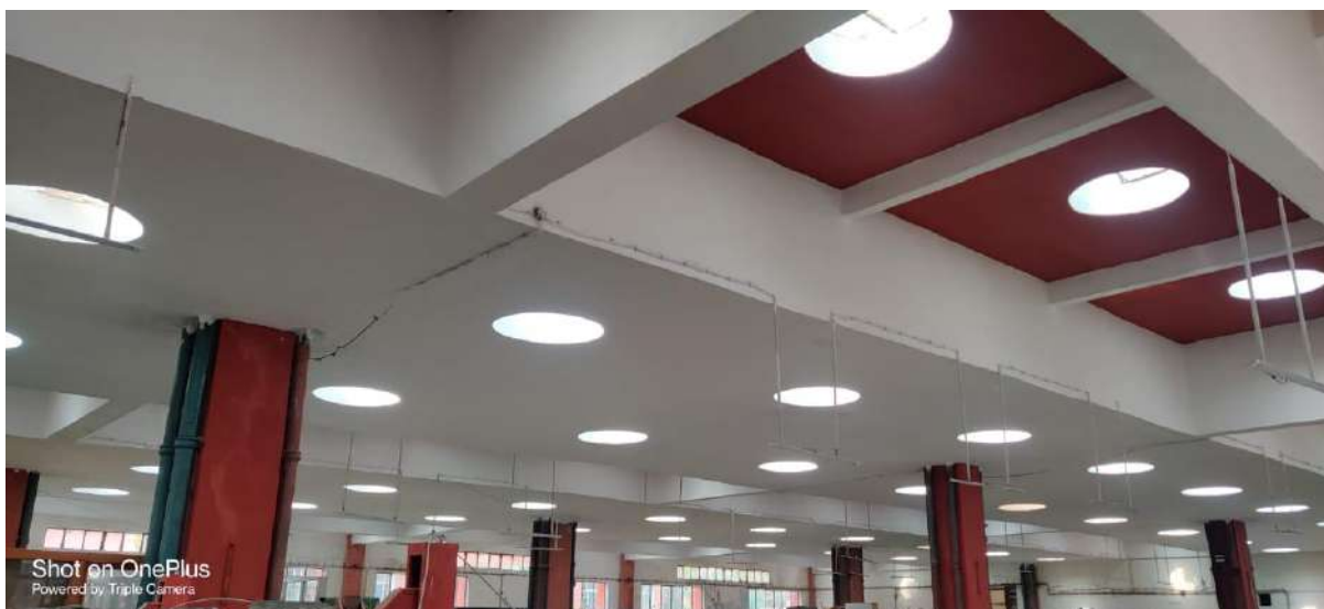
Figure 57: Wall and ceiling paintings on progress.
