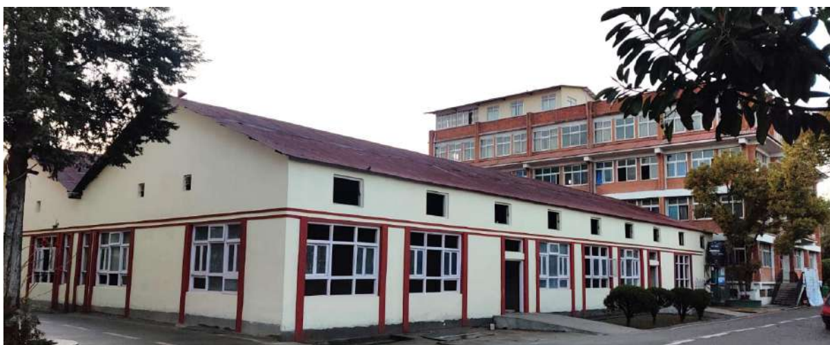
Figure 55: D-block post renovation (ongoing).
