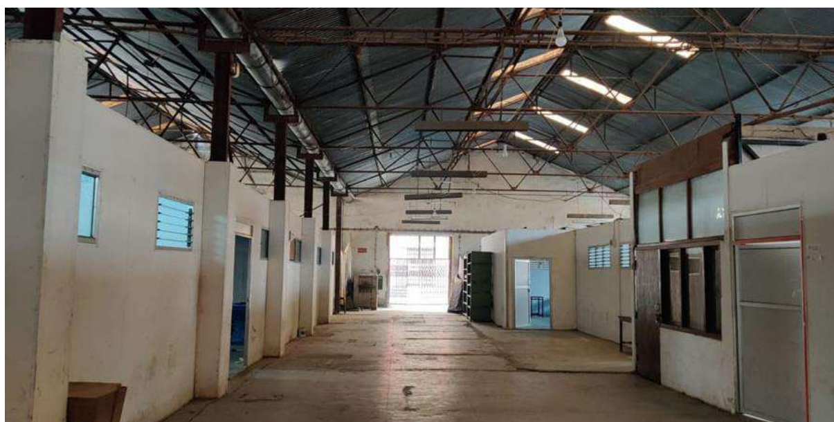
Figure 53: D block prior to renovation.
