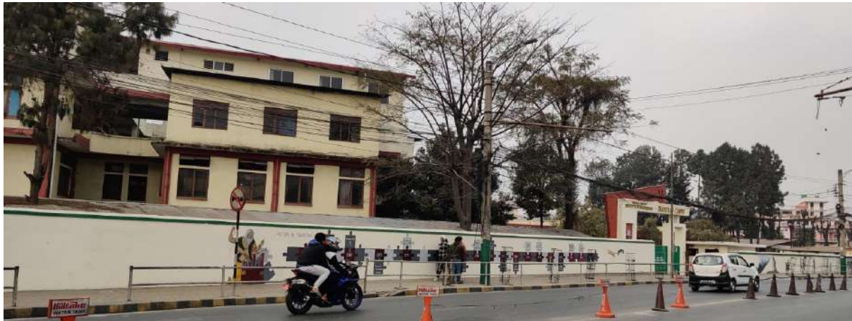
Figure 47: Newly rebuilt boundary walls.
