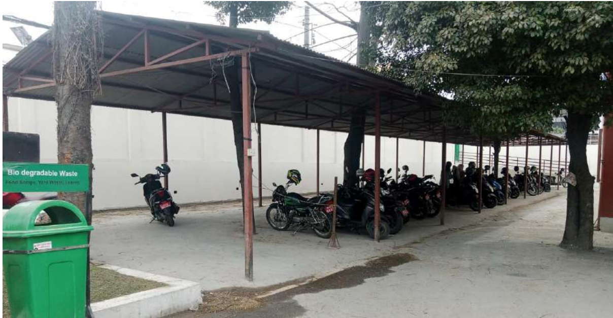
Figure 49: Newly expanded parking space near main entrance.
