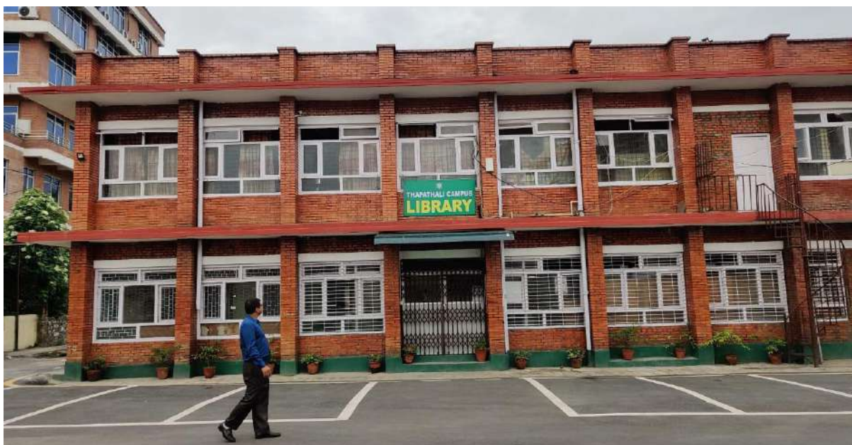
Figure 60: Library after renovation.
