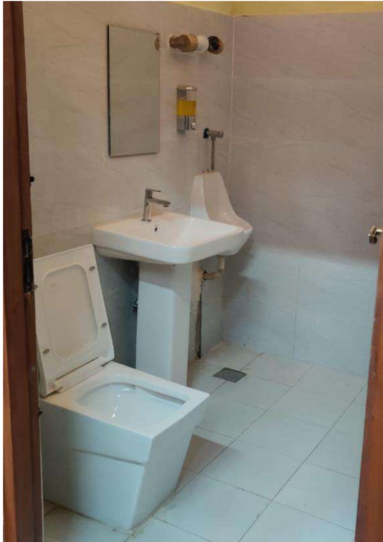
Figure 59: Renovated rest room.
