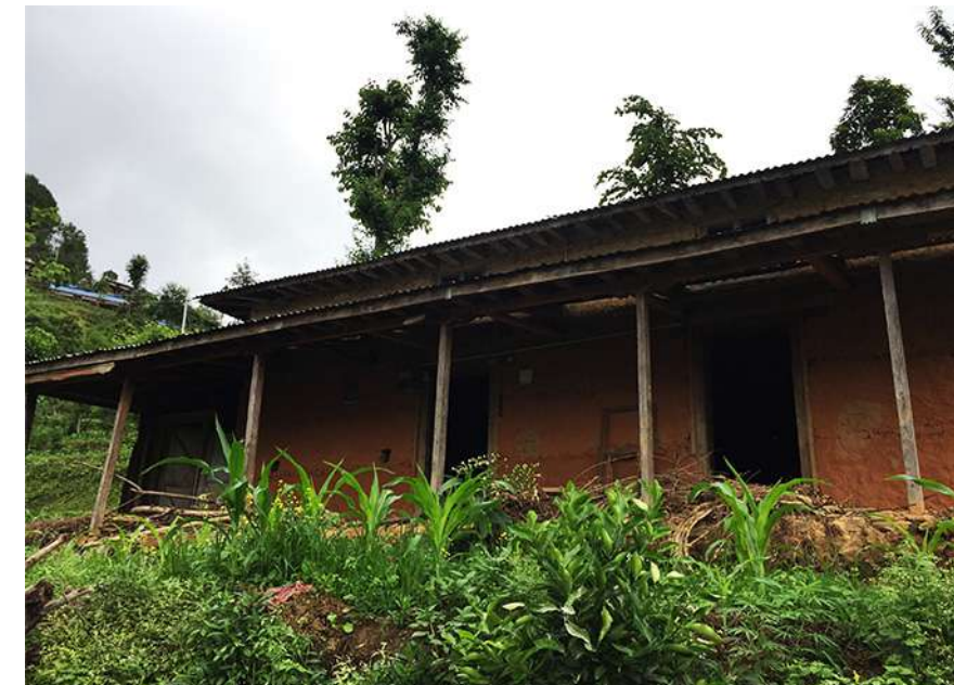
Typical Post-earthquake dwelling, horinzontal support on the wall
