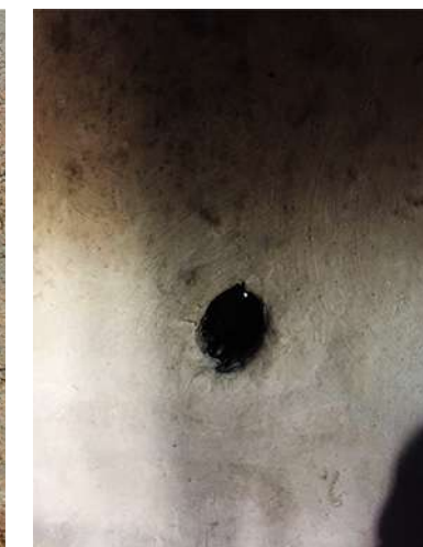
Wall Punctures for Ventilation
