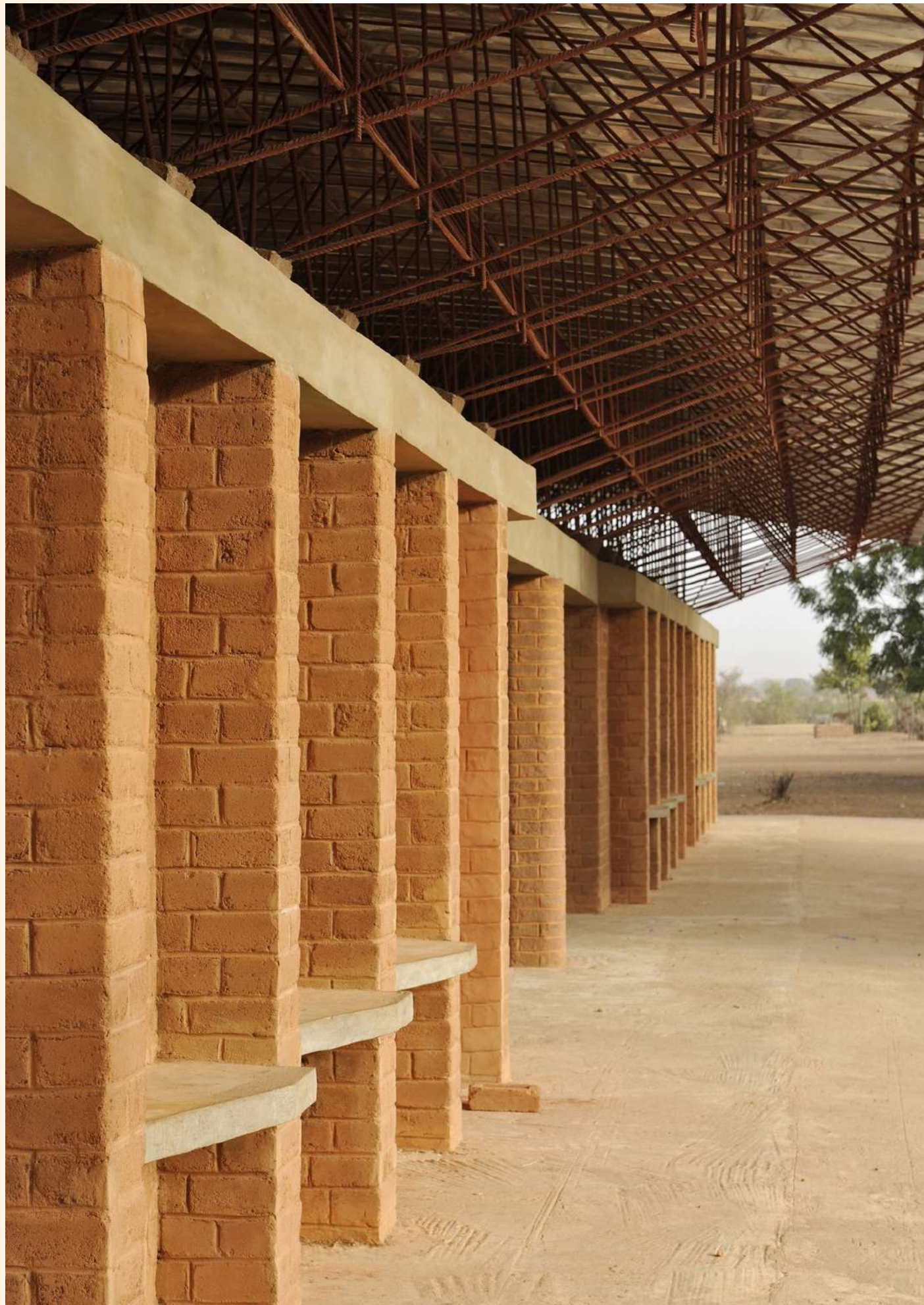
Clay/cement hybrid robust bricks with corrugated metal roof
